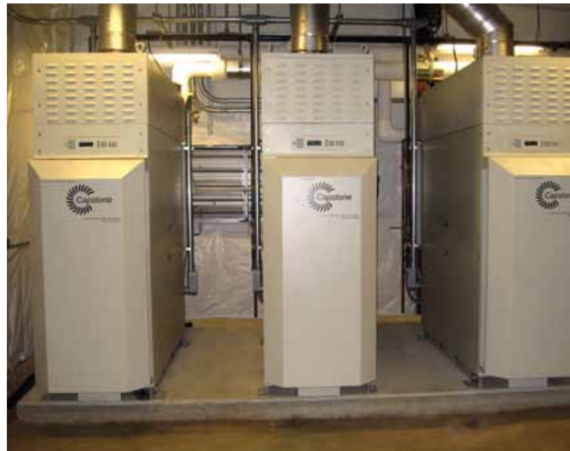
Commissioned in late 2009, the three natural gas C65 ICHP Capstone microturbines produce more than 80 percent of Davidow Hall's electricity and 100 percent of the building's heating and cooling.
